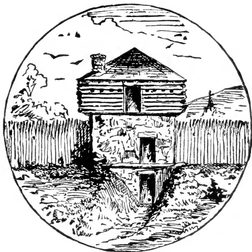
Block House, Built in 1780.
